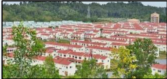
RPN Kampong Tanah Jambu Phase 7
